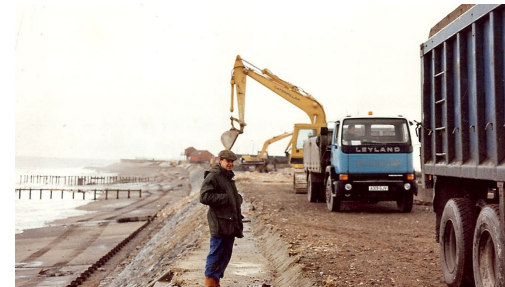
Defence repairs, Chapel St Leonards, 1970s
