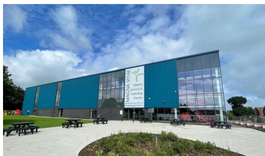
Station Leisure & Learning Centre
