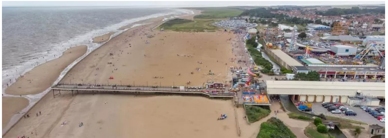
Aerial of Skegness coast featuring the historic Skegness pier in the foreground
