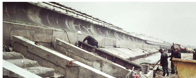
Photo of Sea Defences being built in the 1980s
